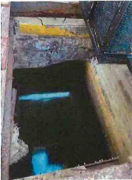
Pump Inlet Points at La Malaria Pump Station After Debris Removal
